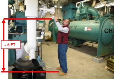
Relocated chiller is 500 tons – allowing for the smallest chiller to remain operating to maximize the free cooling.
